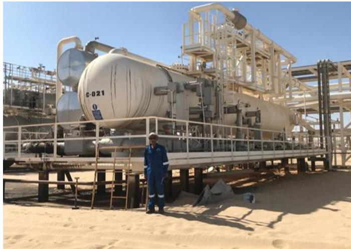
Figure 1. Low Pressure Production Separator C-021 (Personal visit)
